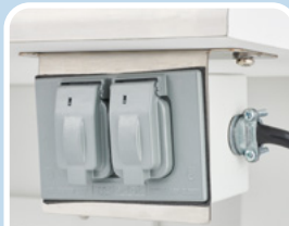
Duplex GFCI Outlets
