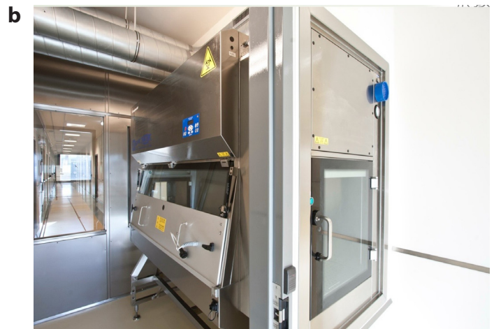
Figure 3. Example of an animal transfer hatch built into a transfer room between the animal barrier and outside.
